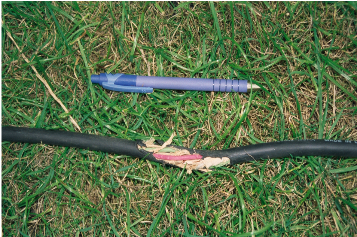
Figure 6-38: Damage to SODAR cabling by rabbits
