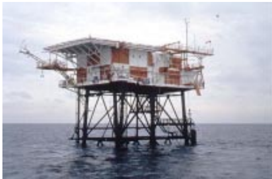
Figure 8: Measuring Post Noordwijk located 9 km off the Dutch coast
